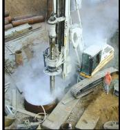
rilled Shafts are deep foundation structural support elements for buildings, bridges, towers, above ground reservoirs or any structure requiring load bearing support. Drilled Shafts range from 12 inches to 10 feet diameter or larger and 5 to 200 feet in depth.
